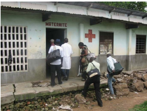
Work has begun to replace the crumbling foundations with a fresh concrete slab.
