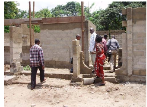
Construction at the Elegance Health Center.
