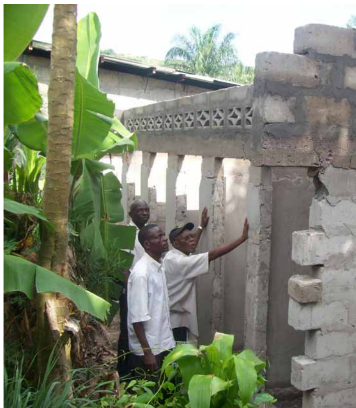
Building the new Community Health Centre in Lemba Imbu, DR Congo.
