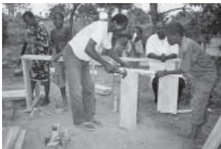
Alabadi School construction, DR Congo
