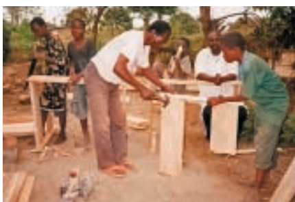
Alabadi School construction, DR Congo
